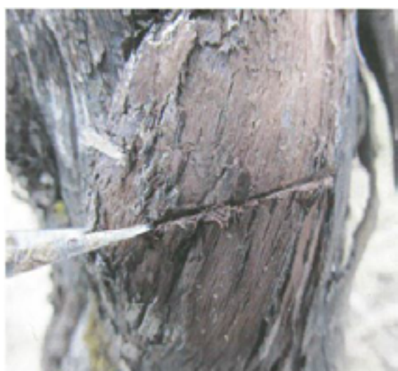
Figure 5: Making a notch (SICAVAC- BIVC)
